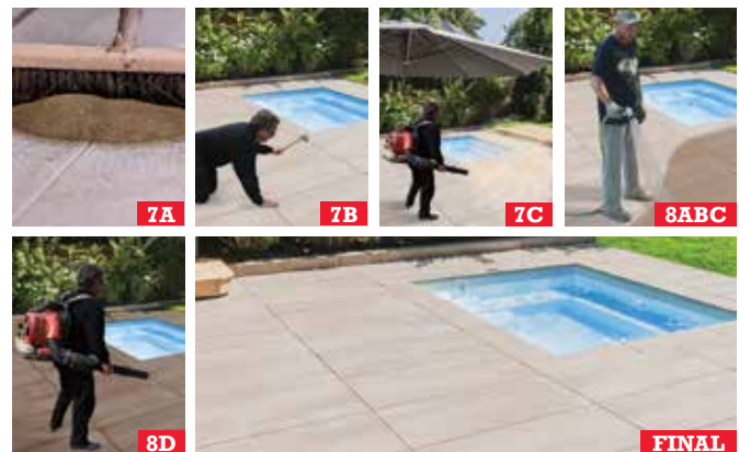
GATOR TILE SAND INSTALLATION STEPS
